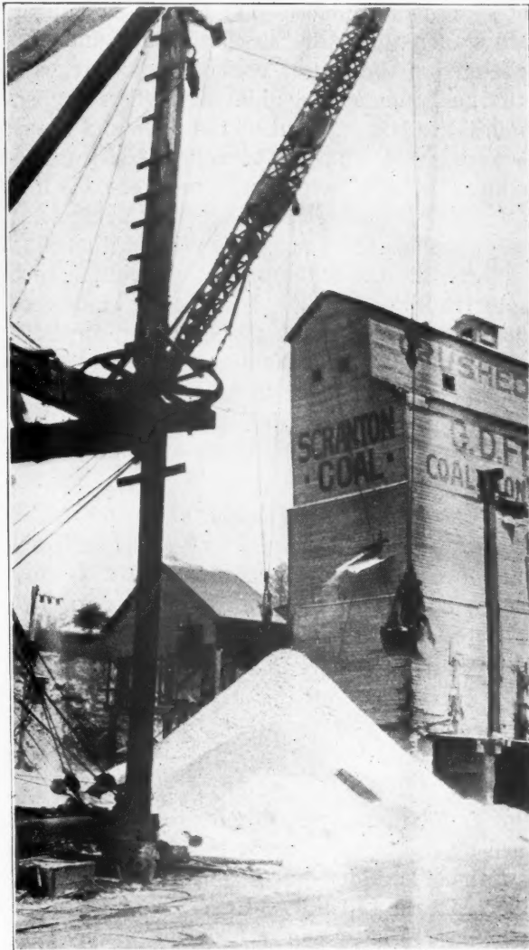
Derrick Handling Crushed Stone to Hoppers
